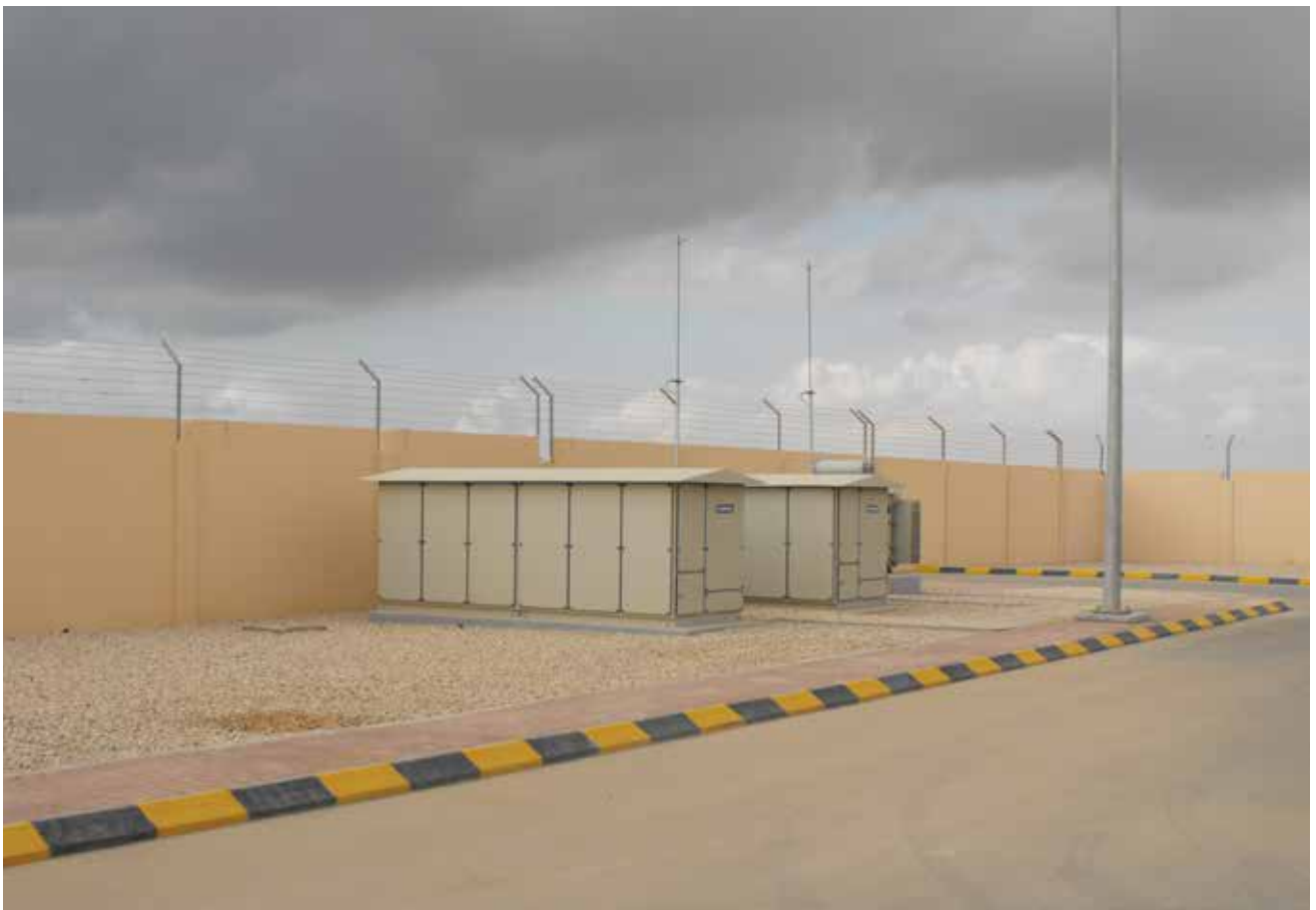
5MVAR 11.5kV Capacitor Bank for DPC, OMAN
