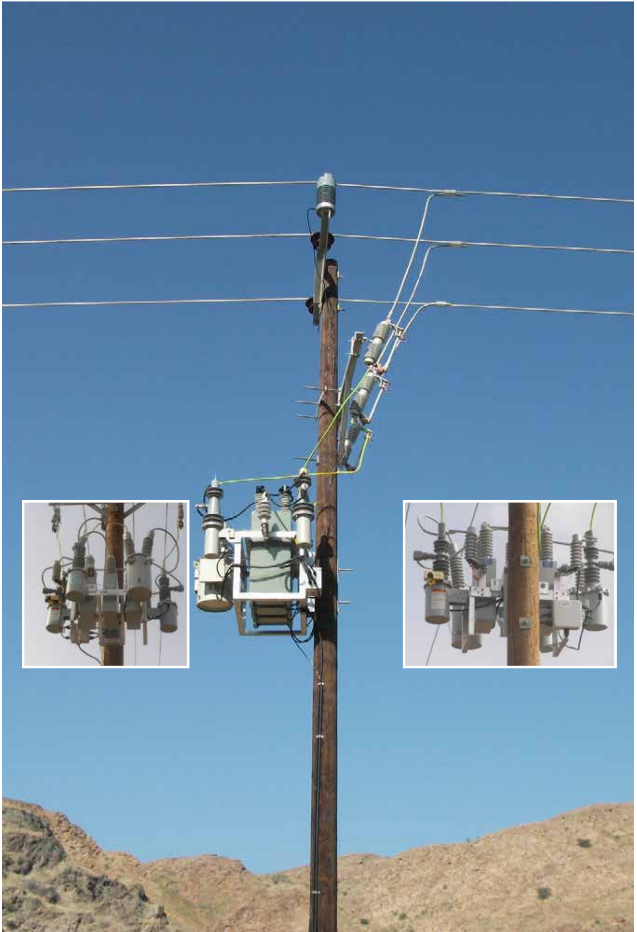
1200KVAR, 11kV Pole Mounted Capacitor Bank at Yiti for MEDC,Oman
