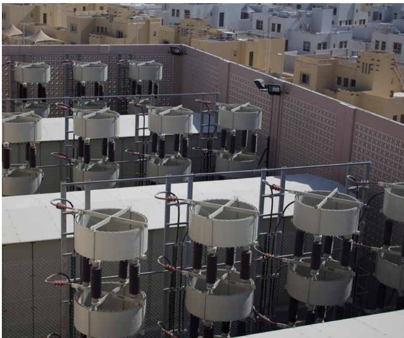
12MVAR, 22kV Detuned Capacitor Bank, Al Falah community project for ADWEA, UAE
