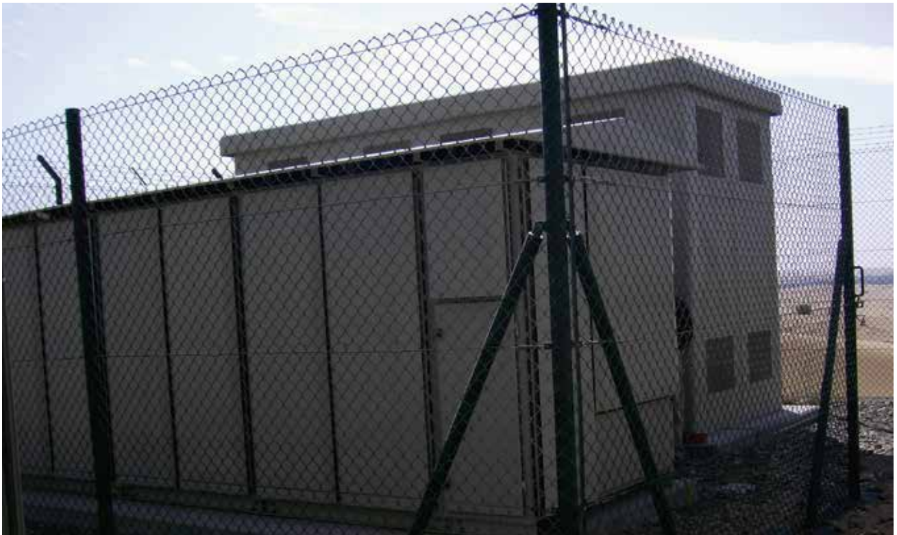
6MVAR, 11kV Detuned Capacitor Bank for ADWEA, UAE
