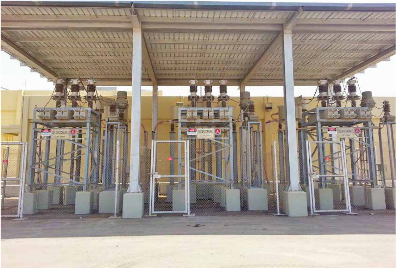
Open execution, 7MVAR @ 13.8kV detuned capacitor bank for SEC, KSA
