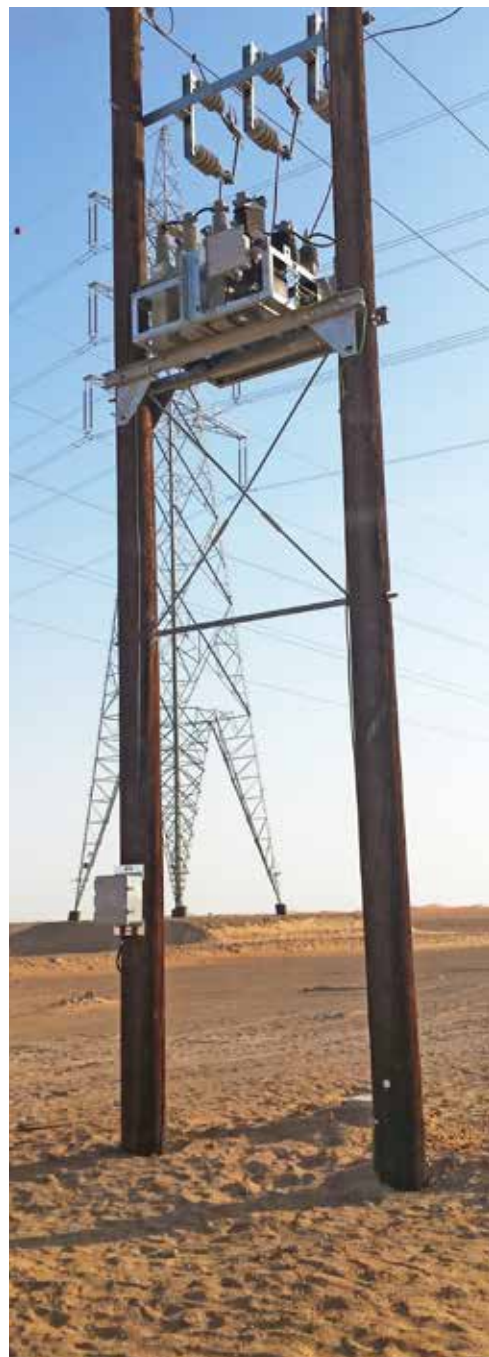
Pole mounted, 600kVAr @ 11kV capacitor bank for AADC, UAE
