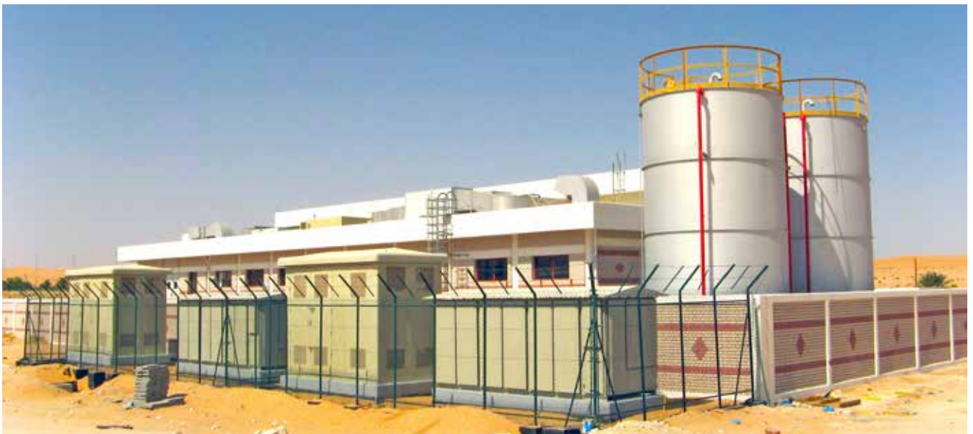
Outdoor metal enclosed, 6MVAR @ 11kV detuned capacitor bank for ADDC, UAE
