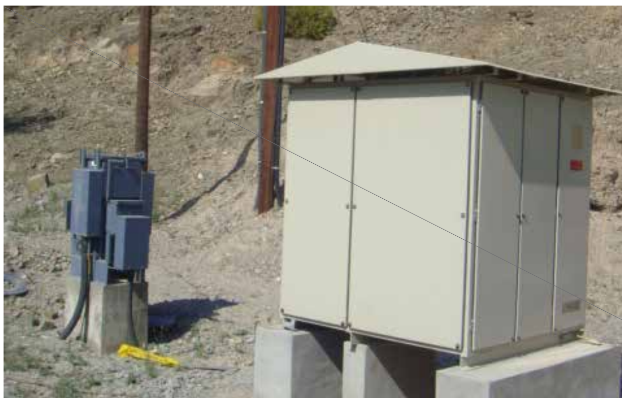
Padmounted 12kV, 0.75MVAR @ 11kV, switched capacitor bank in overhead line distribution network
