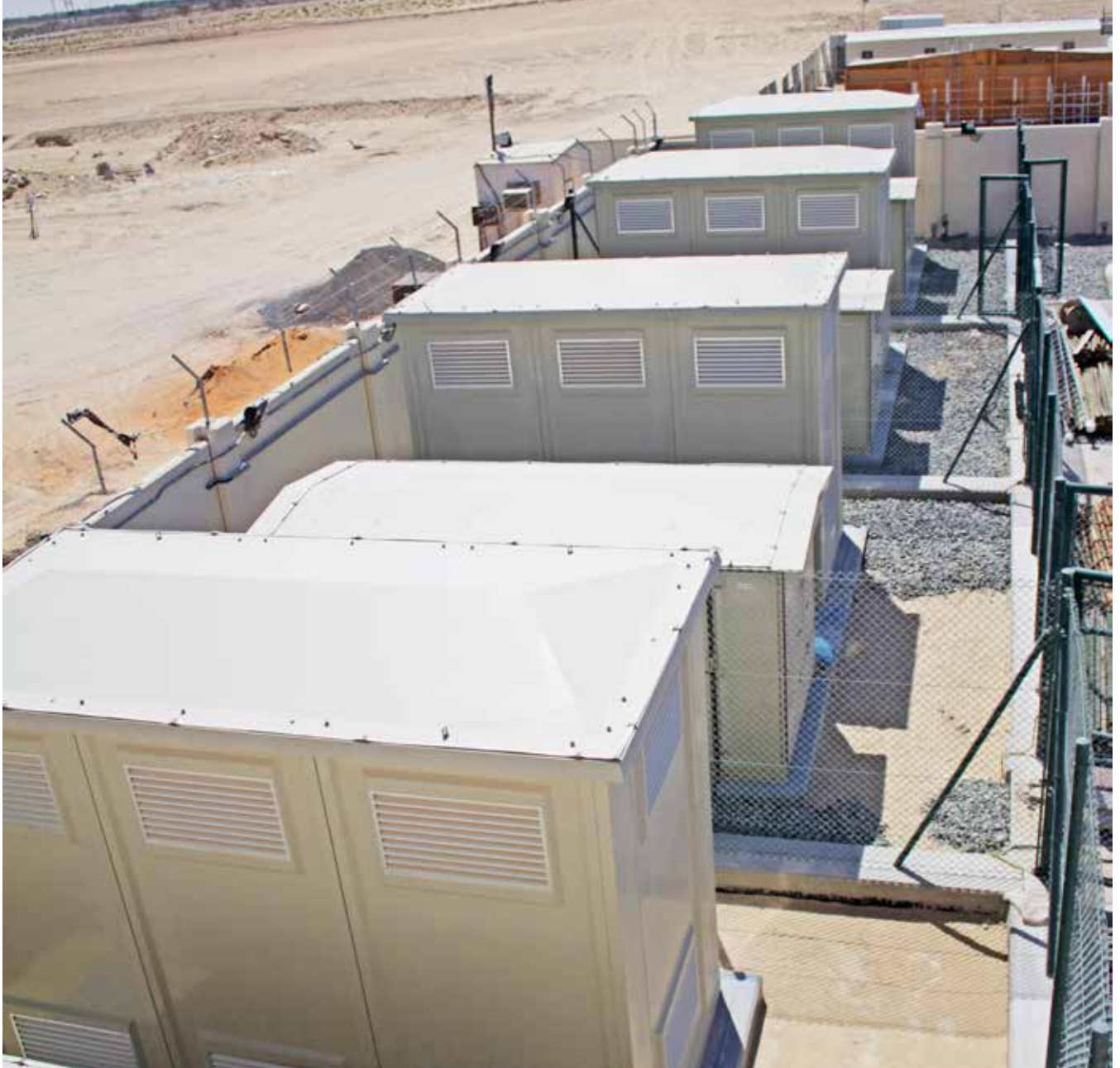
Outdoor metal enclosed, 6MVAR @ 11kV detuned capacitor bank for ADPC, UAE
