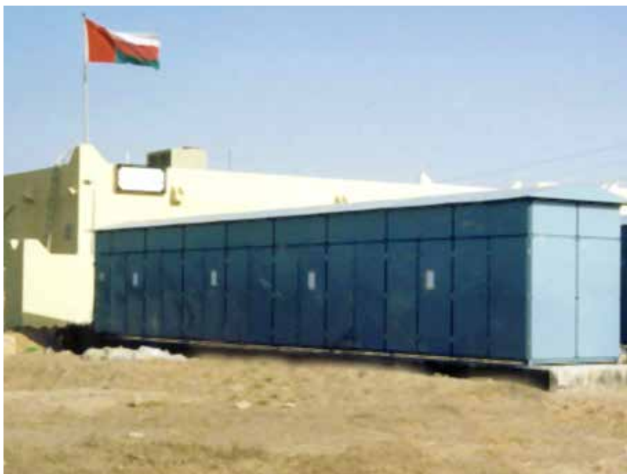
Outdoor metal enclosed, 20MVar @ 33kV detuned capacitor bank for OETC, Oman
