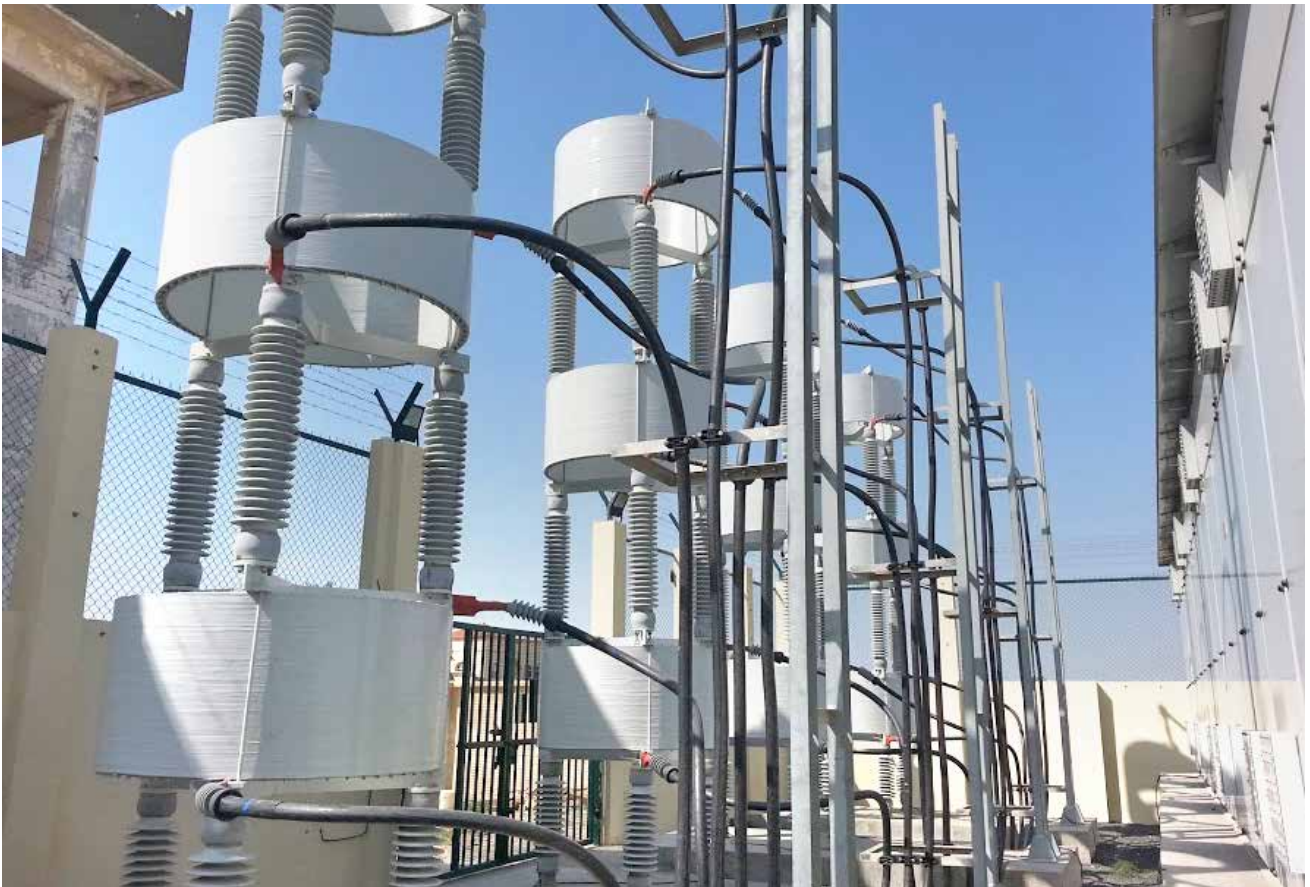
Outdoor metal enclosed, 20MVAR @ 33kV detuned capacitor bank for SEWA, UAE
