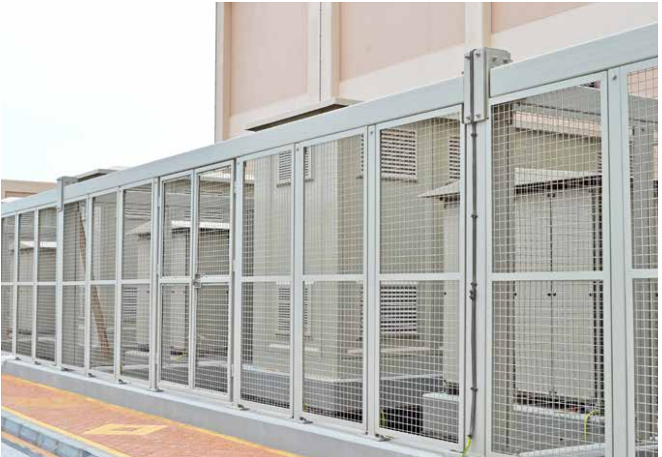
Outdoor metal enclosed, 12MVAR @ 11kV detuned capacitor bank for ADWEA, UAE
