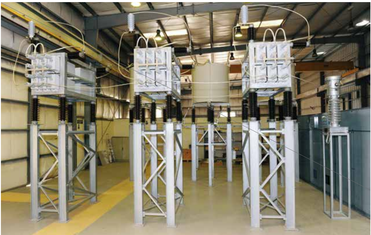
Outdoor 36kV, 20MVar @ 33kV capacitor bank with air core series reactors ready for factory acceptance testing
