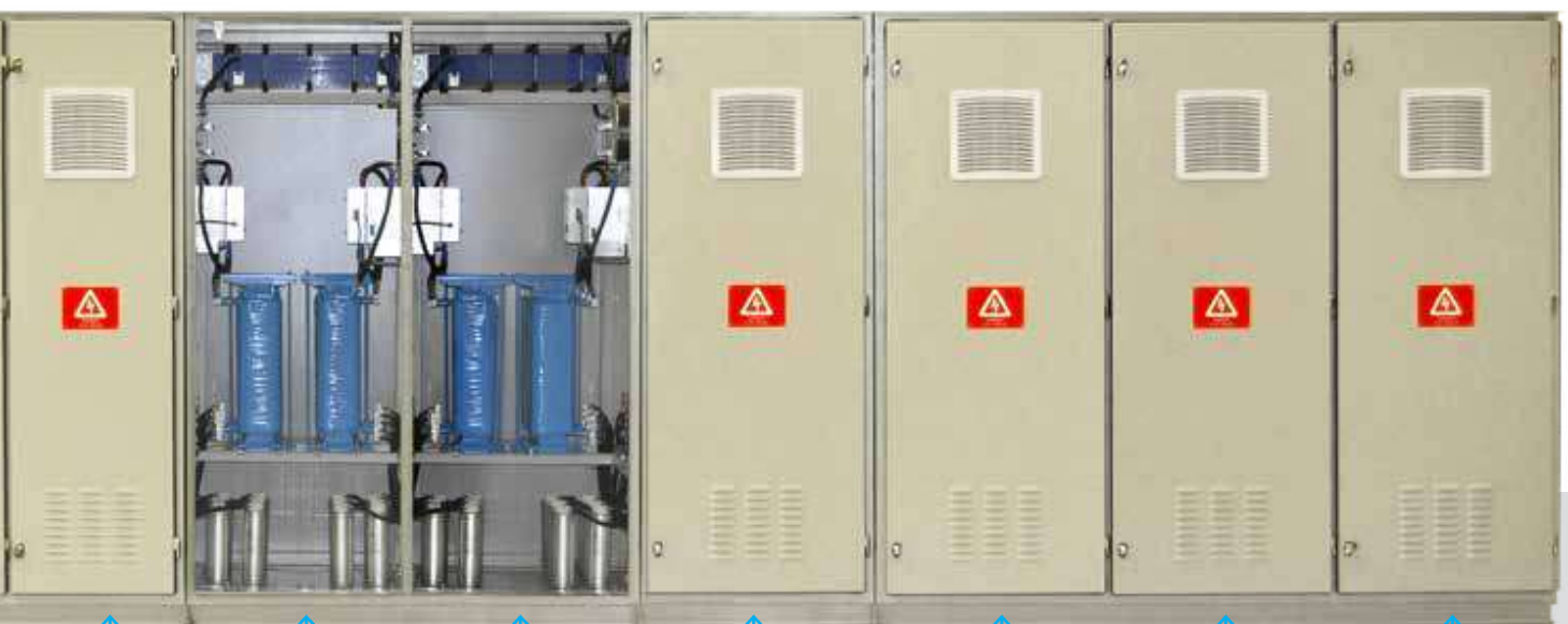
Low voltage thyristor switched 1500kVAr, 14 stage capacitor bank with iron core detuning reactors
