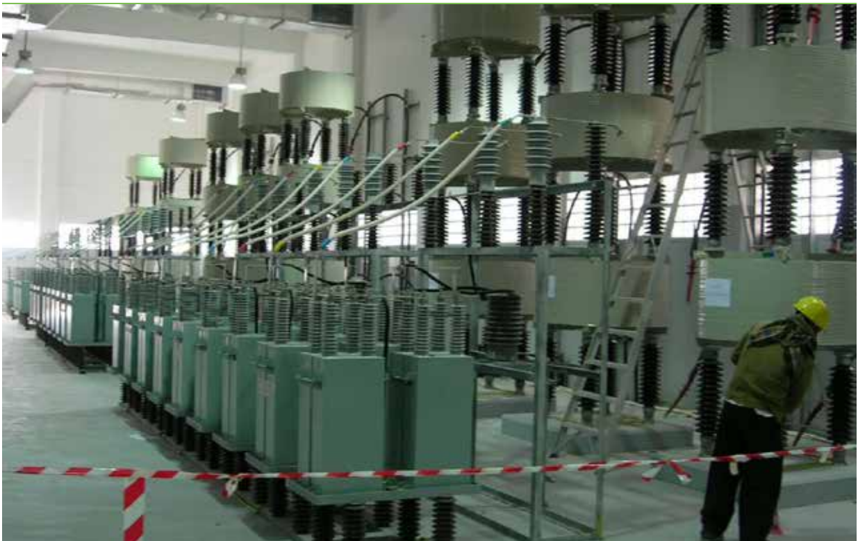
8nos. Indoor 36kV, 5MVAR @ 33kV, capacitor banks with air core series reactors in 220kV/33kV substation.
