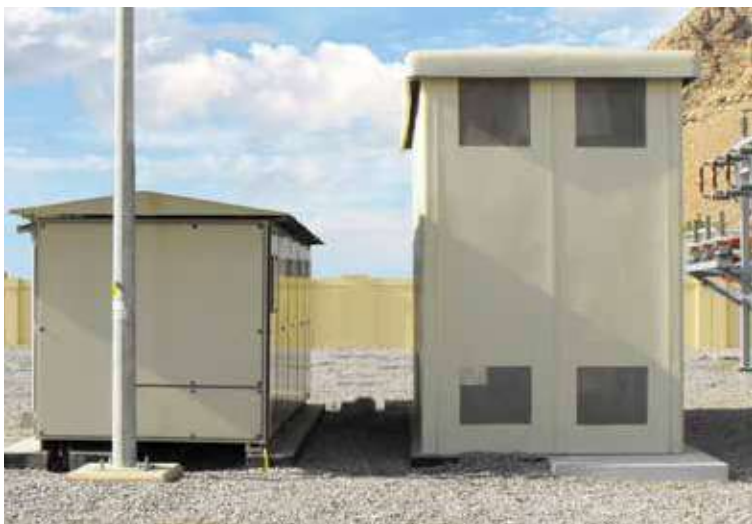
Outdoor metal enclosed, 5MVar @ 11kV detuned capacitor bank for MZEC, Oman
