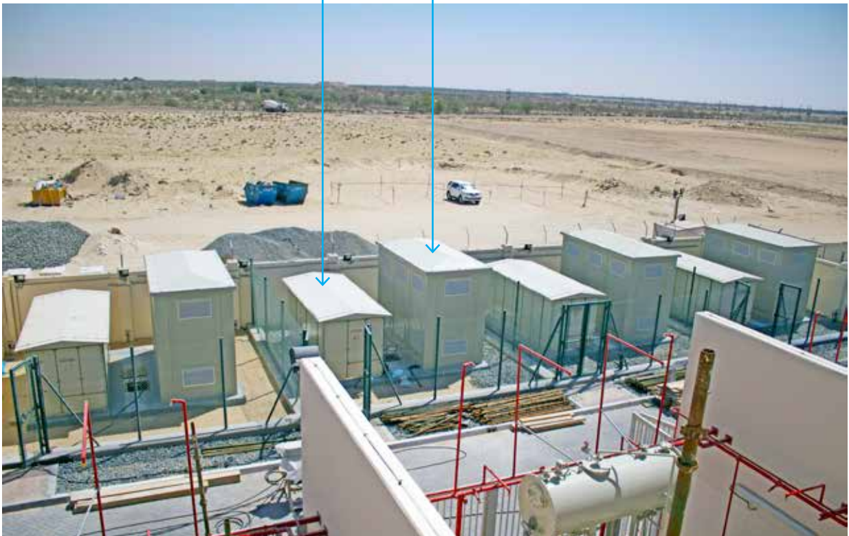
METAL ENCLOSED CAPACITOR BANK
