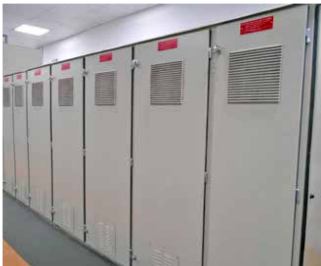
Indoor metal enclosed, 1500kVAr, Thyristor switched, LV detuned capacitor bank for Sohar Steel, Oman
