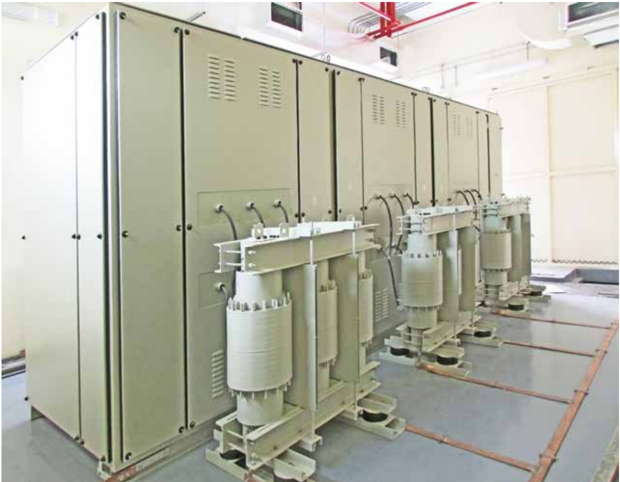
Indoor 12kV, 6MVar @ 11kV multistage switched capacitor bank with iron core series reactor at 33kV/11kV substation
