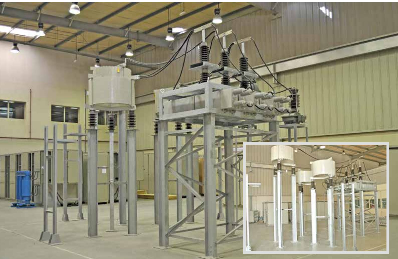
Outdoor 13.8kV, 7MVar capacitor bank with air core series reactors
