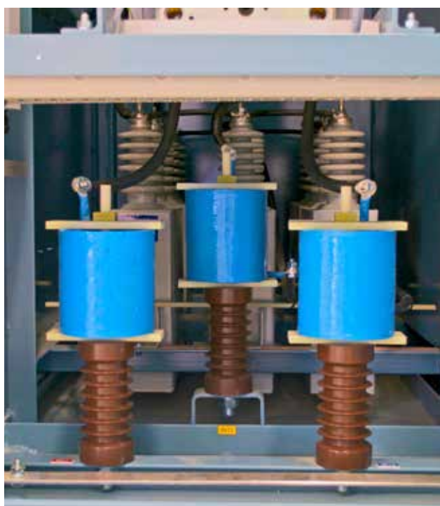
Inrush current limiting reactors
