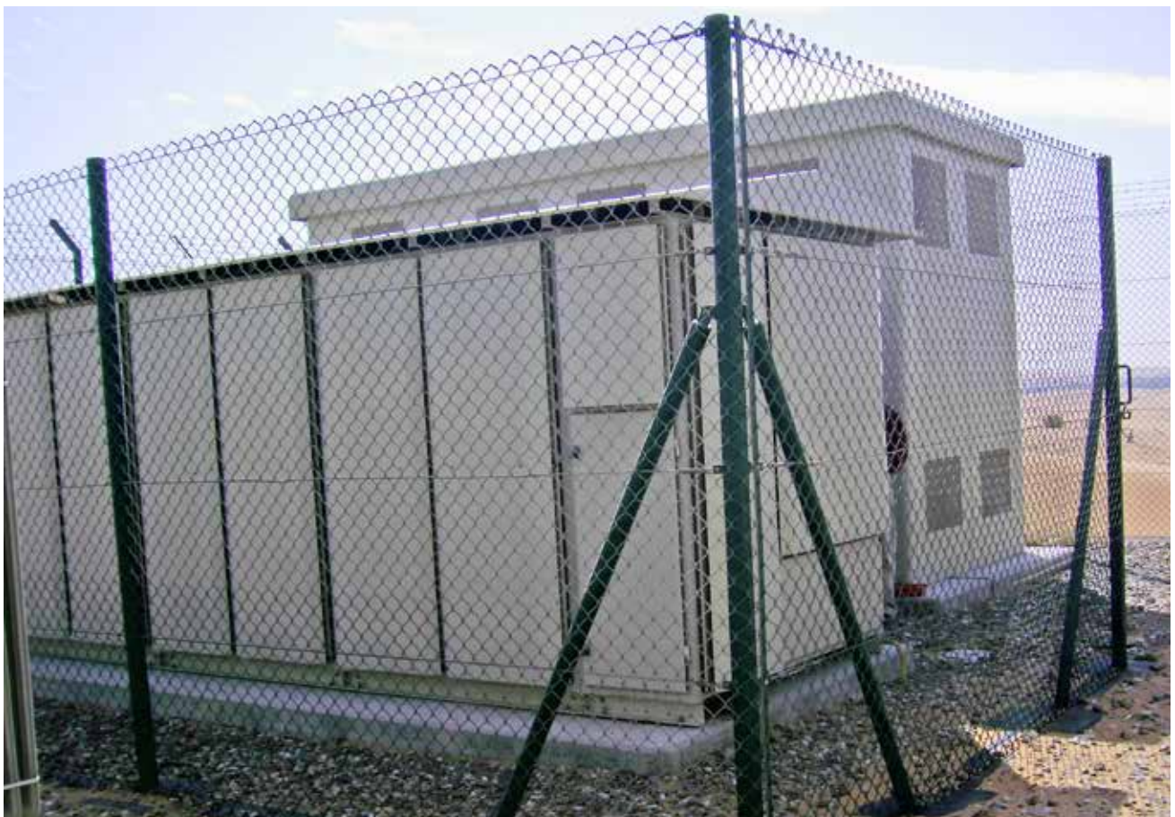
Outdoor metal enclosed, 6MVAR @ 11kV detuned capacitor bank for ADWEA, UAE
