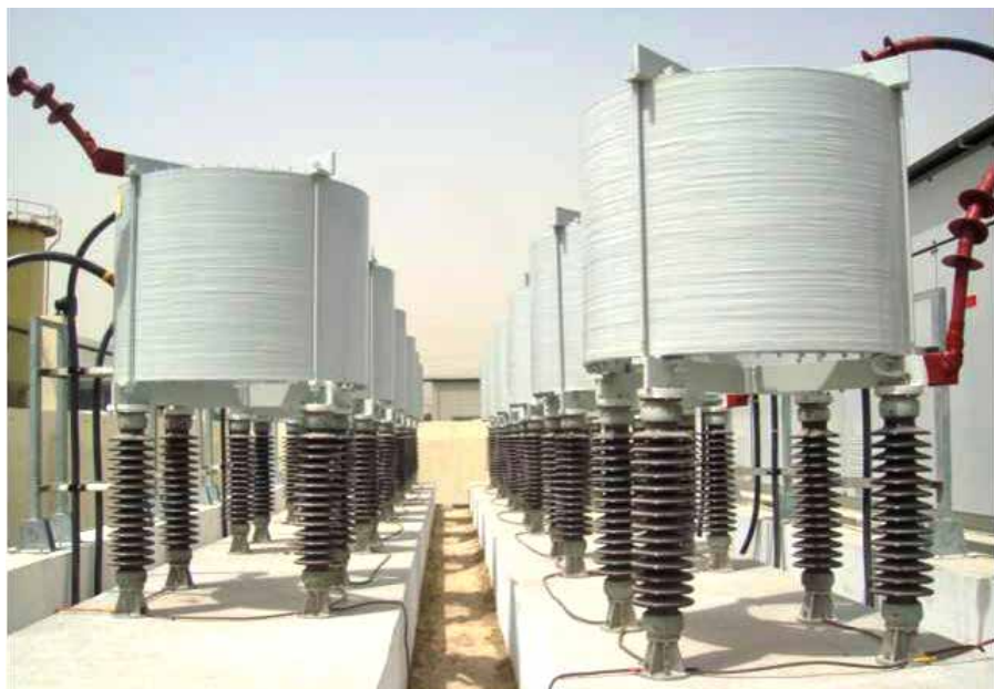
Outdoor 36kV air core detuning reactors for SEWA, UAE
