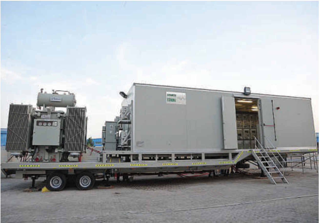
Mobile Package Substation for FEWA
