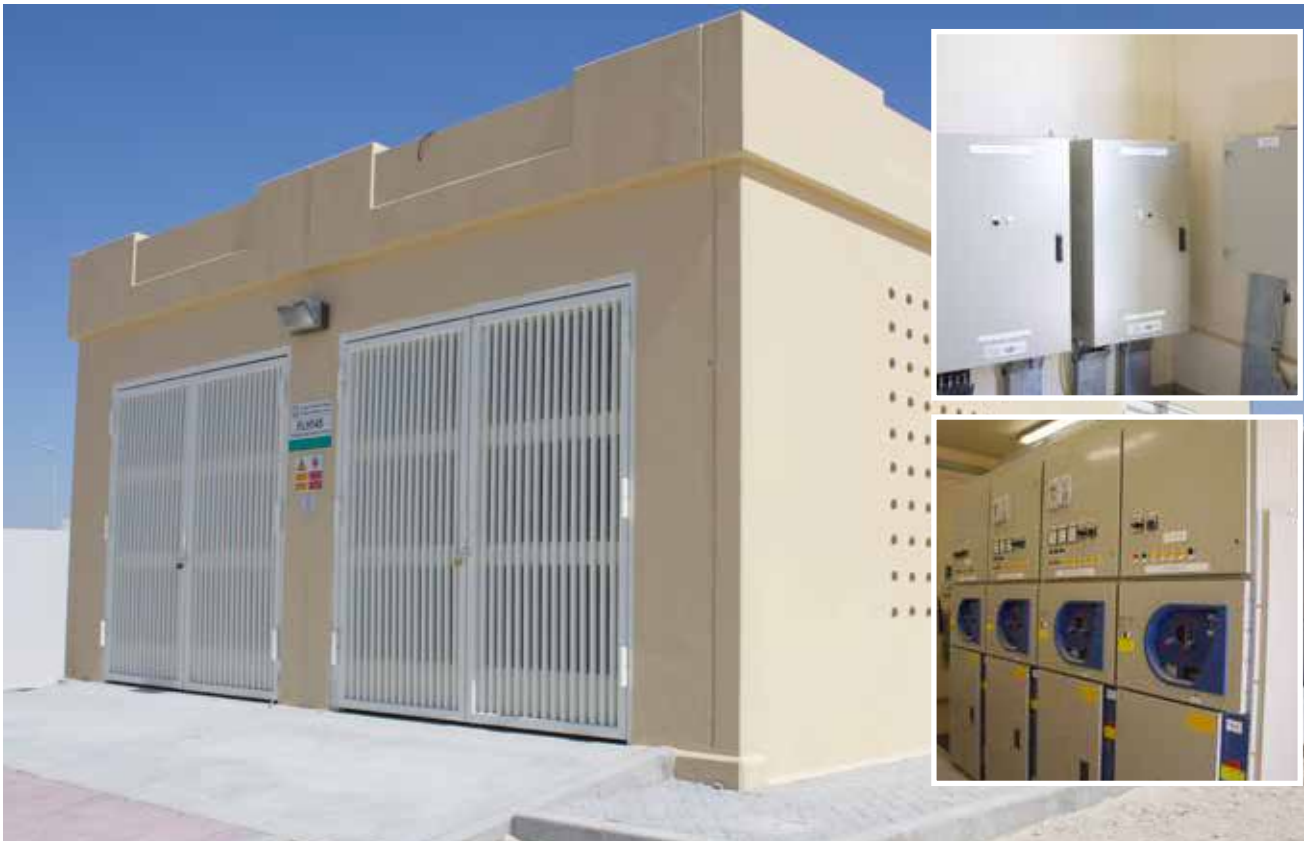
22kV Medium Voltage Switchgear, Al Falah community project for ADWEA, UAE
