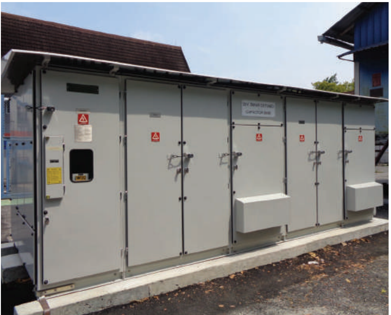
12kV 5MVar Outdoor Capacitor banks with Iron core reactors for TNB, Malaysia
