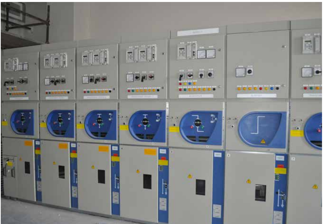
11kV Medium Voltage Switchgear at Deerfield town Square for ADWEA, UAE
