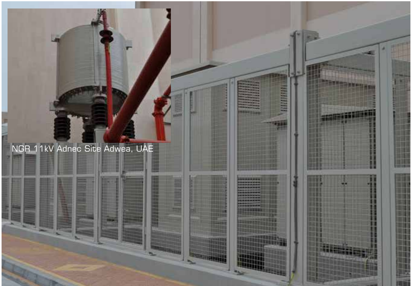
12MVAR, 11kV Detuned Capacitor Bank at ADNEC Site for ADWEA, UAE
