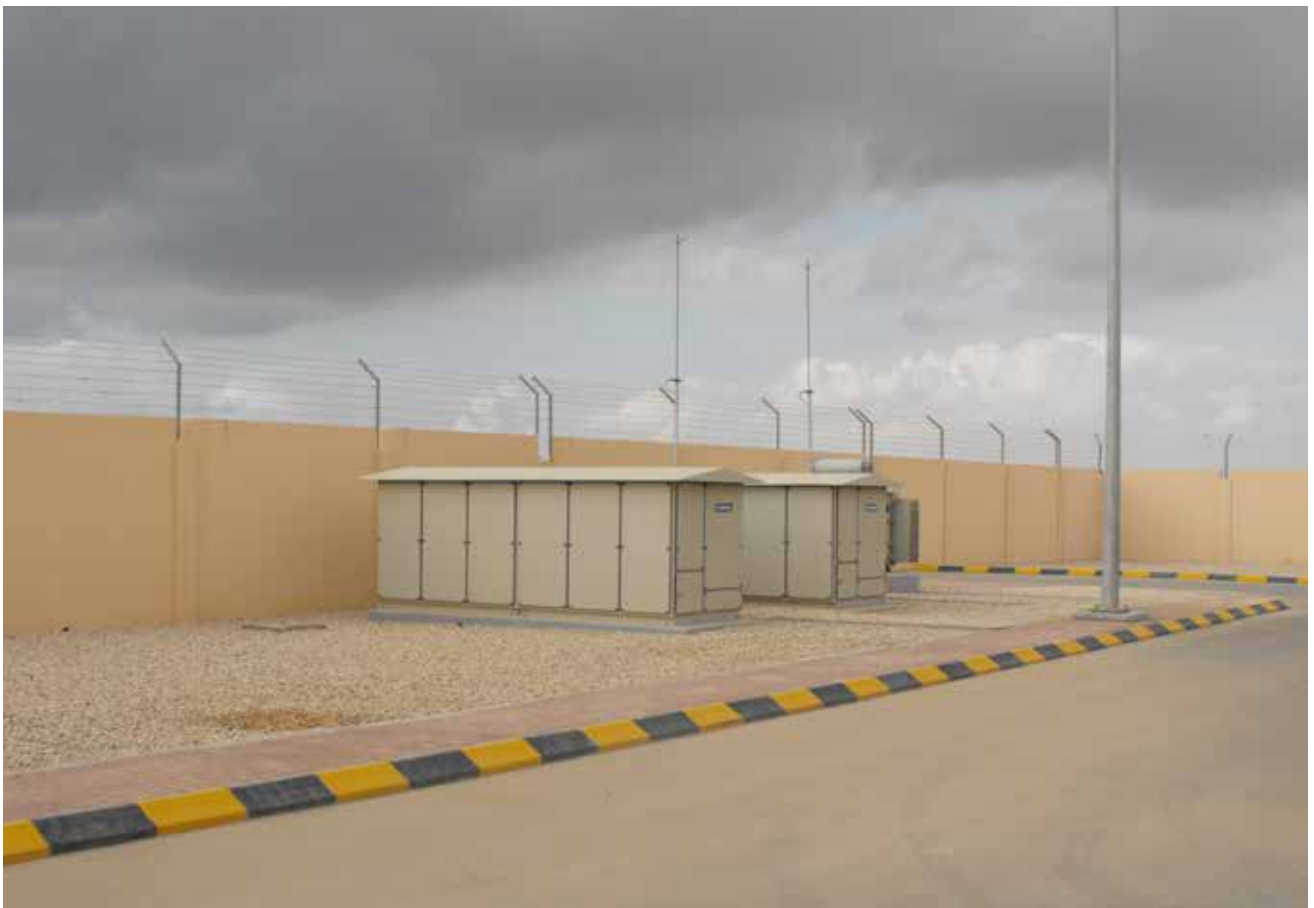
5MVAR 11.5kV Capacitor Bank for DPC, OMAN
